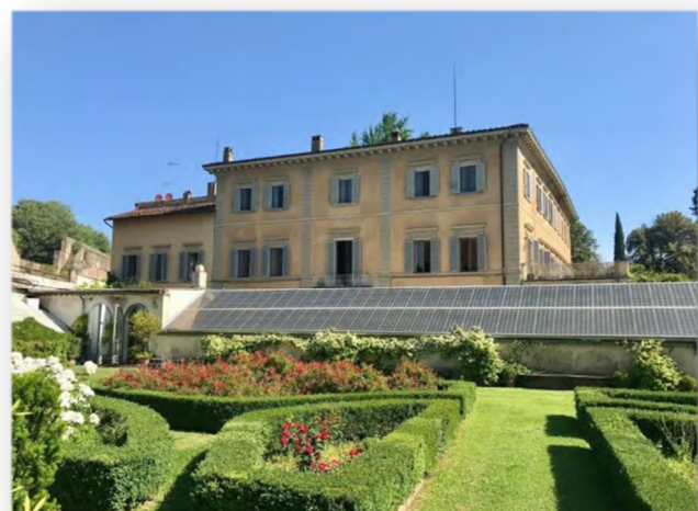
Photovoltaic greenhouse in the Torrigiani Garden in Florence
